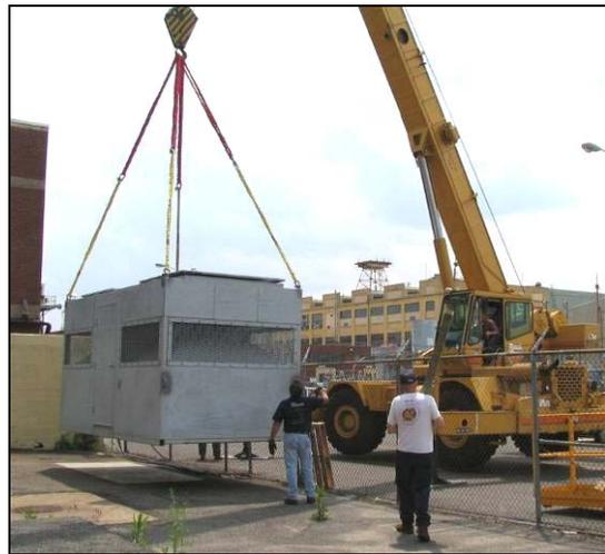
**Figure 9. Positioning 3.5 MW resistor load bank for higher power Static Load tests**
